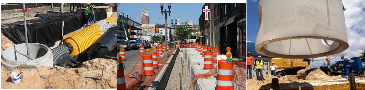
Figure 18: Typical green-gray infrastructure construction (Source: Tetra Tech, 2017)
