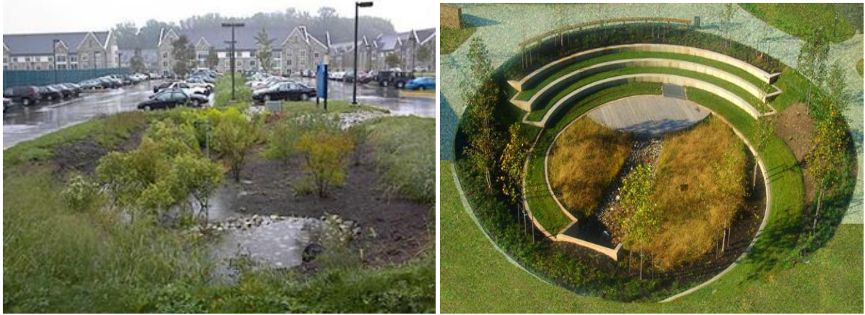
Figure 14: Typical surface infiltration basins (Source: Tetra Tech, 2017).
